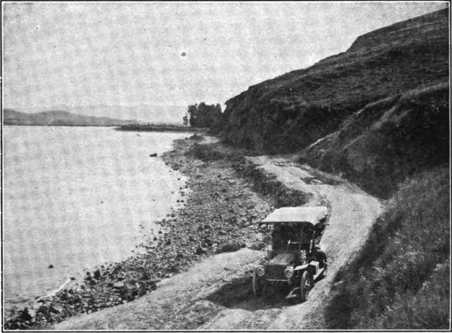
ON THE BAY SHORE ROAD, ALONG THE ROUTE OF THE RAILWAY CUT-OFF LINE
